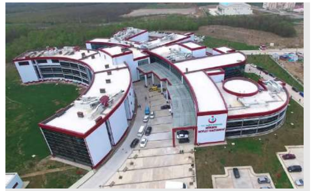
Hendek State Hospital Sakarya
