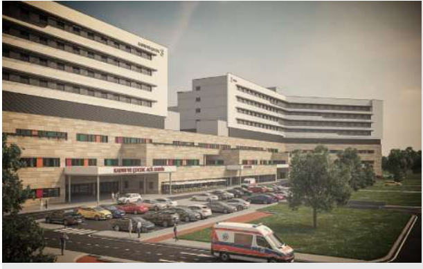
Bursa City Hospital Bursa
