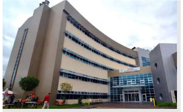
Devrek State Hospital Zonguldak
