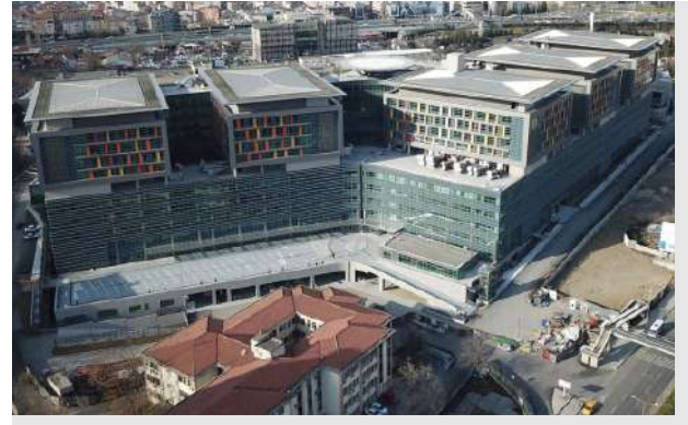
Okmeydanı Research and Training Hospital İstanbul
