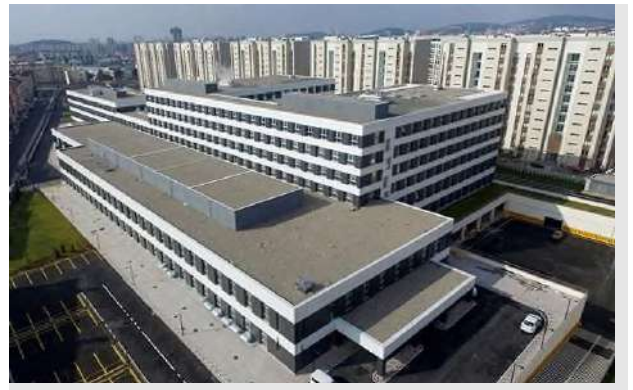
Sancaktepe State Hospital İstanbul
