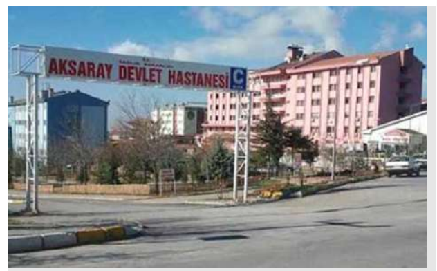
Aksaray State Hospital Aksaray
