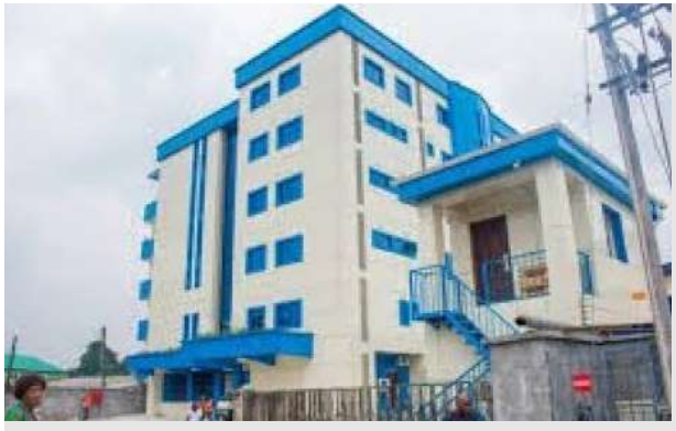
Princess Medical Center Port Harcourt Nigeria
